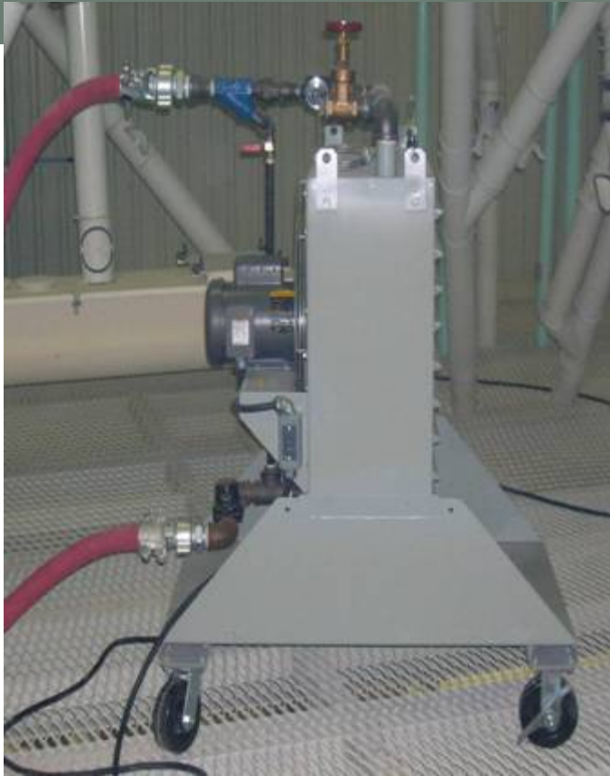
Armstrong International Inc Mill 3, June 2006
